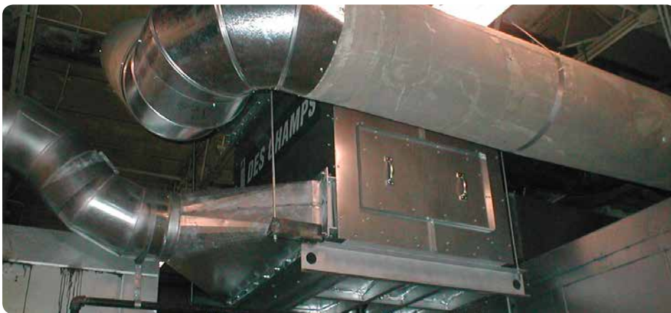
Munters installed two Z-Duct Series 85 heat exchangers for the paint curing process to take the exhaust air as waste heat and use it to pre-heat make-up air instead.
